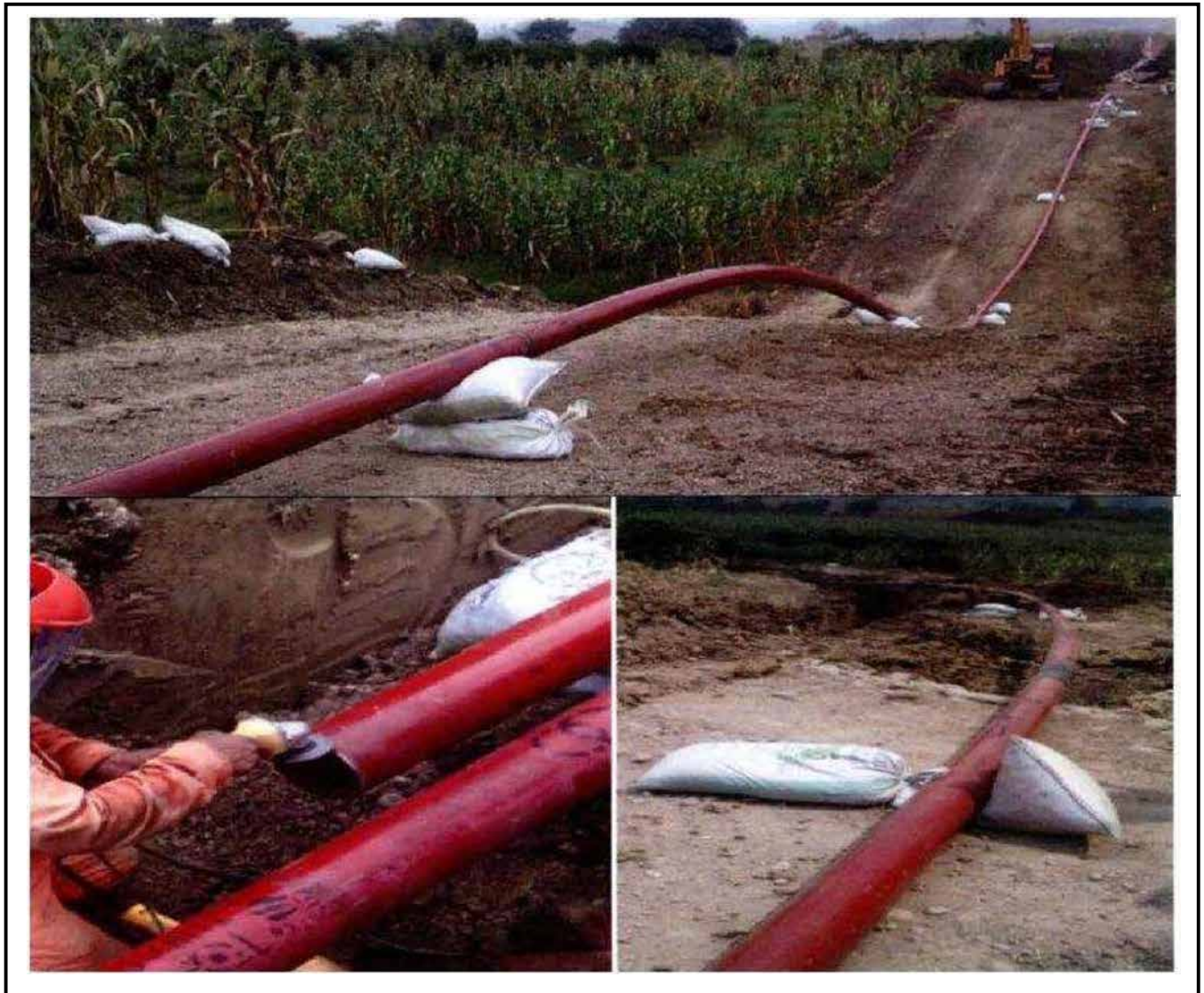
Fig. 6 Construction of a 6-5/8 Ø x 0.600 km Oil Pipeline
