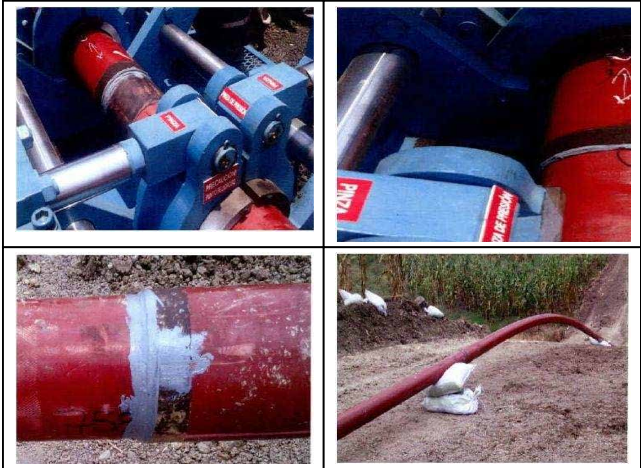
Fig. 5 Fabrication of a mechanical joint using SURE-LOCK
